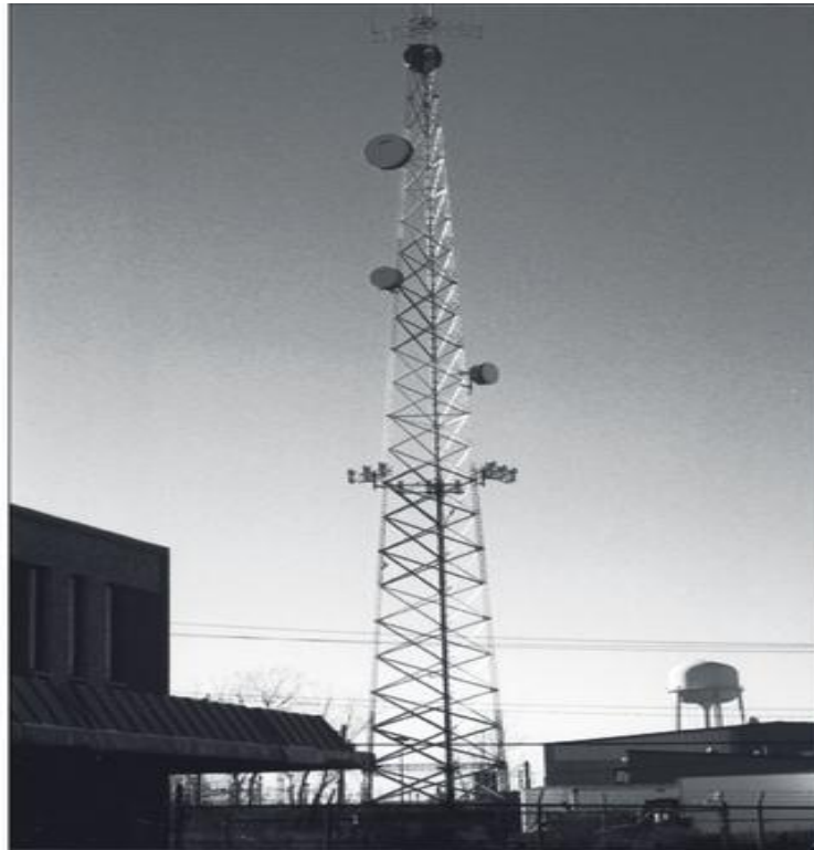
Figure 3-11 A typical microwave tower and antenna
